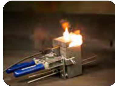
Step 5: Reaction is made, open mold to remove connection and clean mold before next connection.
